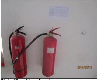
Photo of fire safety equipment fire extinguishers.JPG
