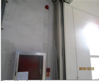
Photo of fire safety equipment fire alarm.JPG
