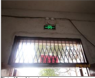
Photo of fire safety equipment fire exit sign and emergency light.JPG
